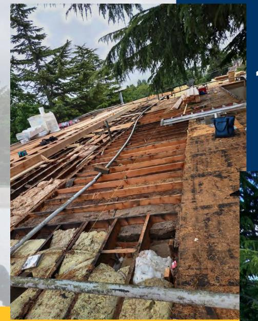
9,000 Square Feet Apartment Building Remove existing Built-up Roof System and Decking Eliminate Insulation and CompleteVentilation Correction Install Stick Frame Tapered System to Eliminate Standing Water Install 60 Mil TPO Roof Membrane
